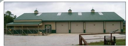
Reg. Pole Frame Buildings Are Heavy 29 Ga. Metal, Three 2"x6" T&G Splashboards, All Poles 5"x5" Or Larger, CCA Treated, Fully Trimmed With One 3'x6' Walk-Through Door & One Large Sliding Door.
