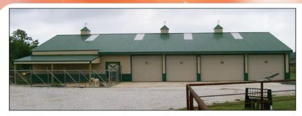
Reg. Pole Frame Buildings Are Heavy 29 Ga. Metal, Three 2"x6" T&G Splashboards, All Poles 5"x5" Or Larger, CCA Treated, Fully Trimmed With One 3'x6' Walk-Through Door & One Large Sliding Door.
