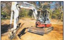
Takeuchi TB153FR Excavator
