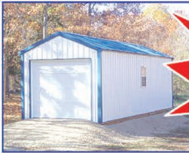
Portable Garage on Gravel Pad
