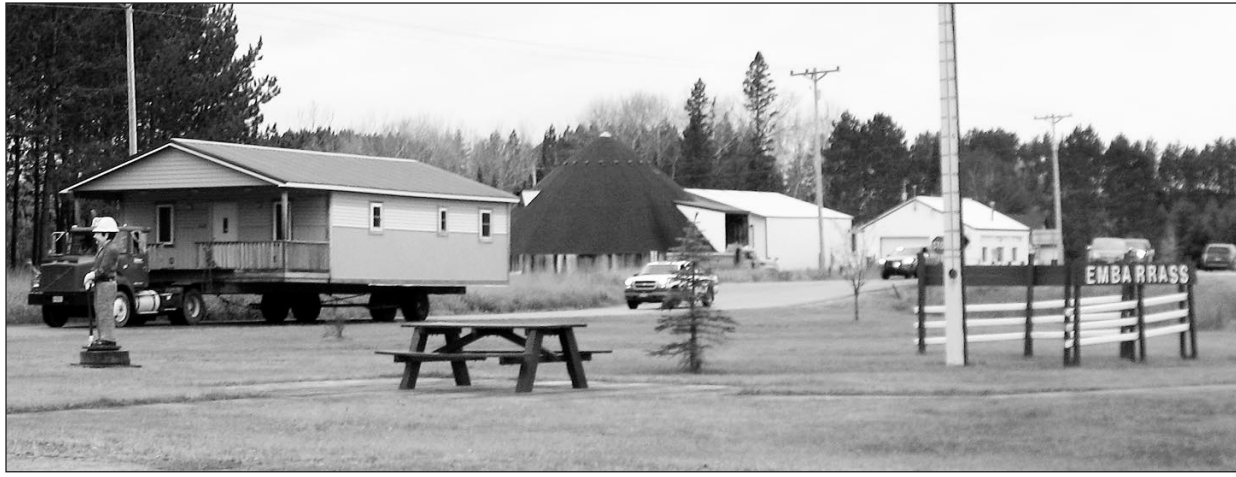
The new Embarrass Post Office building was moved to its Hwy. 21 site on Saturday. C&C Winger has been working on the project. The U.S. Postal Service will soon be coming in to take over interior renovations. The opening date is still a few months away. The township would like to thank the IRRRB for help with funding for this project. submitted photo
