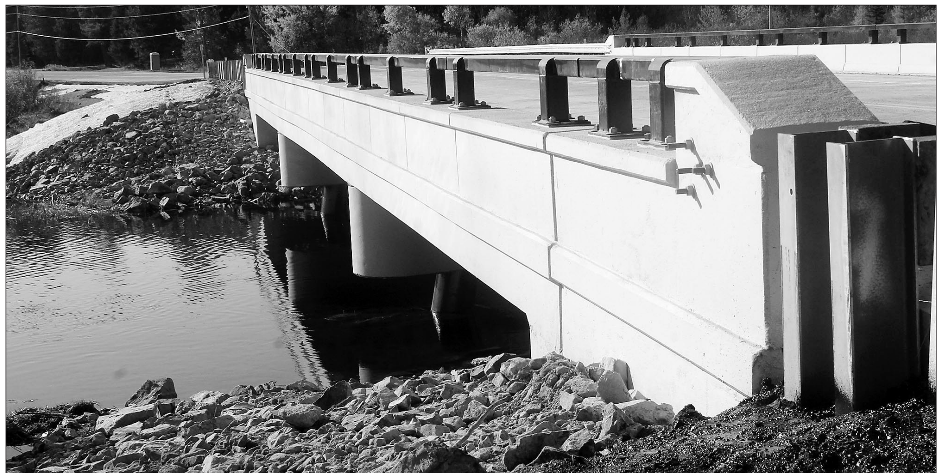
The new bridge on County State Aid Highway 88 (Grant McMahan Boulevard) west of Ely opened last Friday. The bridge and road will need to re-close next spring, scheduled for May 21 to June 9, for the final road paving, marking and shouldering, and bridge painting. photo by K. Vandervort
