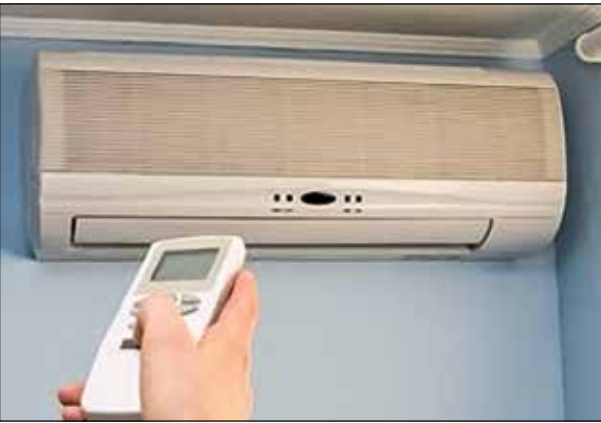
The mini-split unit, or “head” is installed on an indoor wall. They can be operated by remote controllers.
