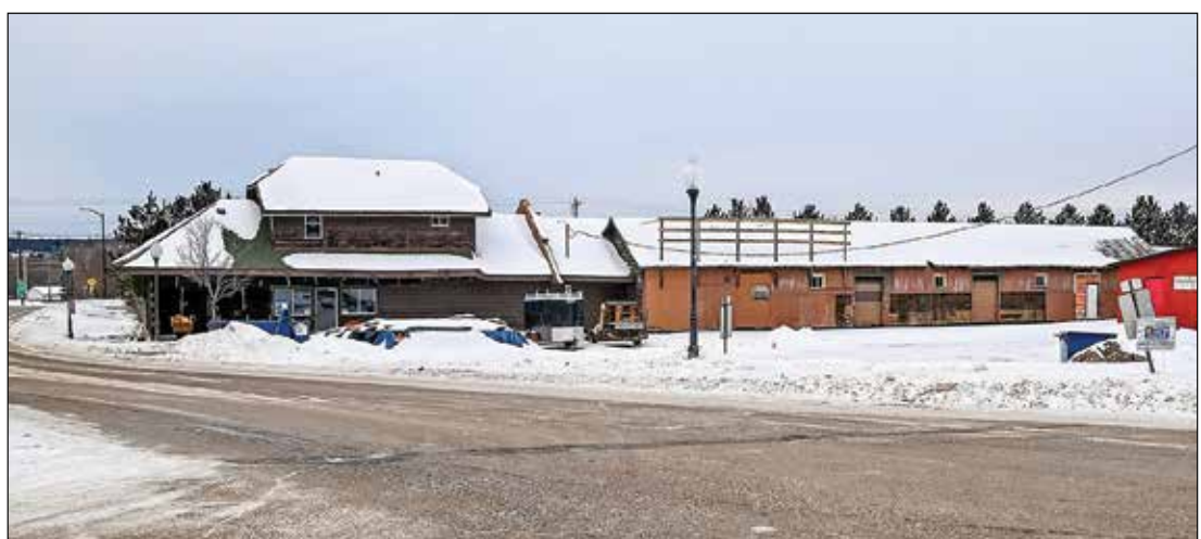
Ely's former railroad depot, which was most recently used by an outfitter. photo by C. Clark
