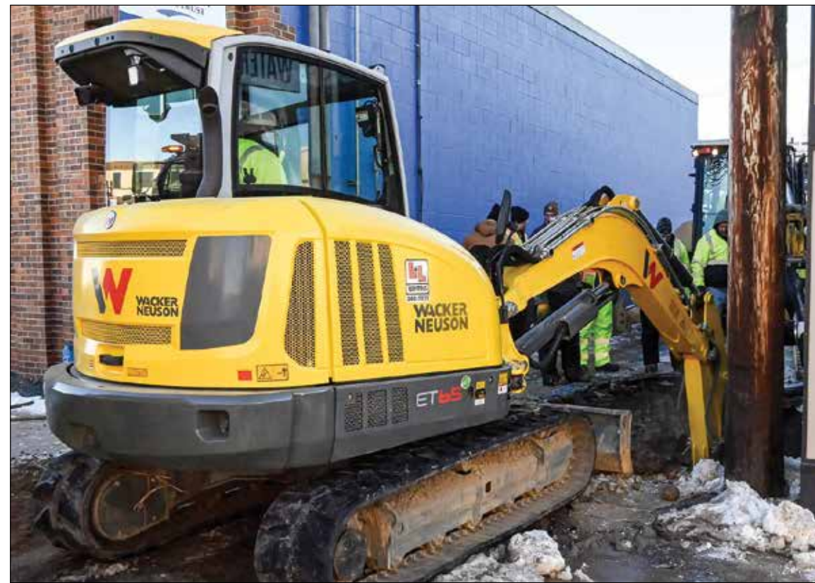
A crew from the Ely Public Works Department excavating where a brass fitting failed at the junction of the water main and a water service line in the alley behind the James Drug building, now the home to Potluck Kitchenware. photo by C. Clark
