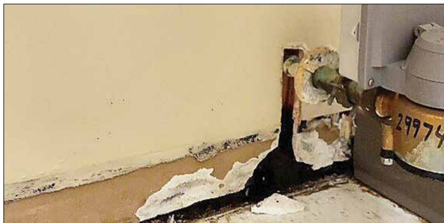
Above: The club paid to have the leaking water pipe inside a wall of the large single room space they lease. Left: Mold damage in the drywall was present throughout their leased space. submitted photos
