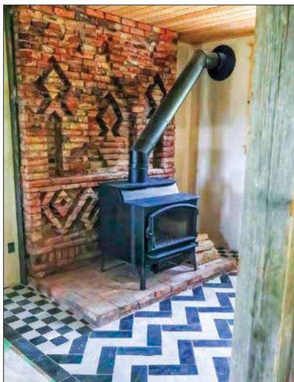
A soft woodfired brick wall installation carved in a traditional Yemeni style yaagur pattern was shipped to the U.S. in three pieces.
