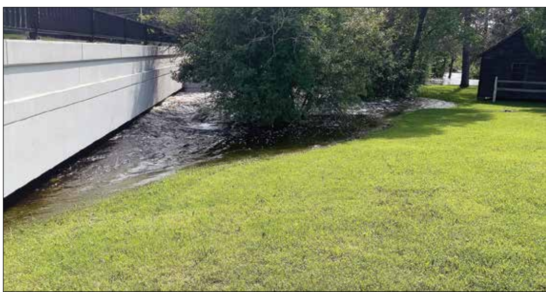
The path to the start of the Ancient Cedars Trail was totally submerged (swimmable if you were a dog!). The waters did recede by early last week and the boardwalk was not damaged, but some of the support beams floated away and will need replacing. The trail is open, but please walk with care. East Two River was licking the bottom of the bridge by the old Iron Ore Bar and overflowed its banks into the mini-park picnic area.
