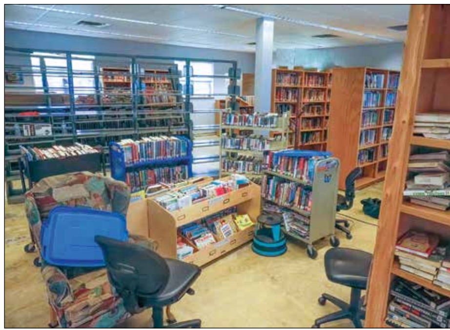
A sticky tile floor, carts of books and empty shelves are all signs of the volunteer response to the six inches of water that seeped into the building during the flood. Removing the waterlogged carpet quickly was essential for protection the library's collection. photo by D. Colburn
