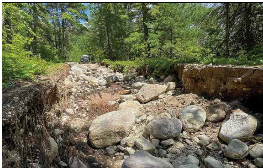
Left: A boat landing access road at Big Lake, north of Ely, was washed away down to boulders.
