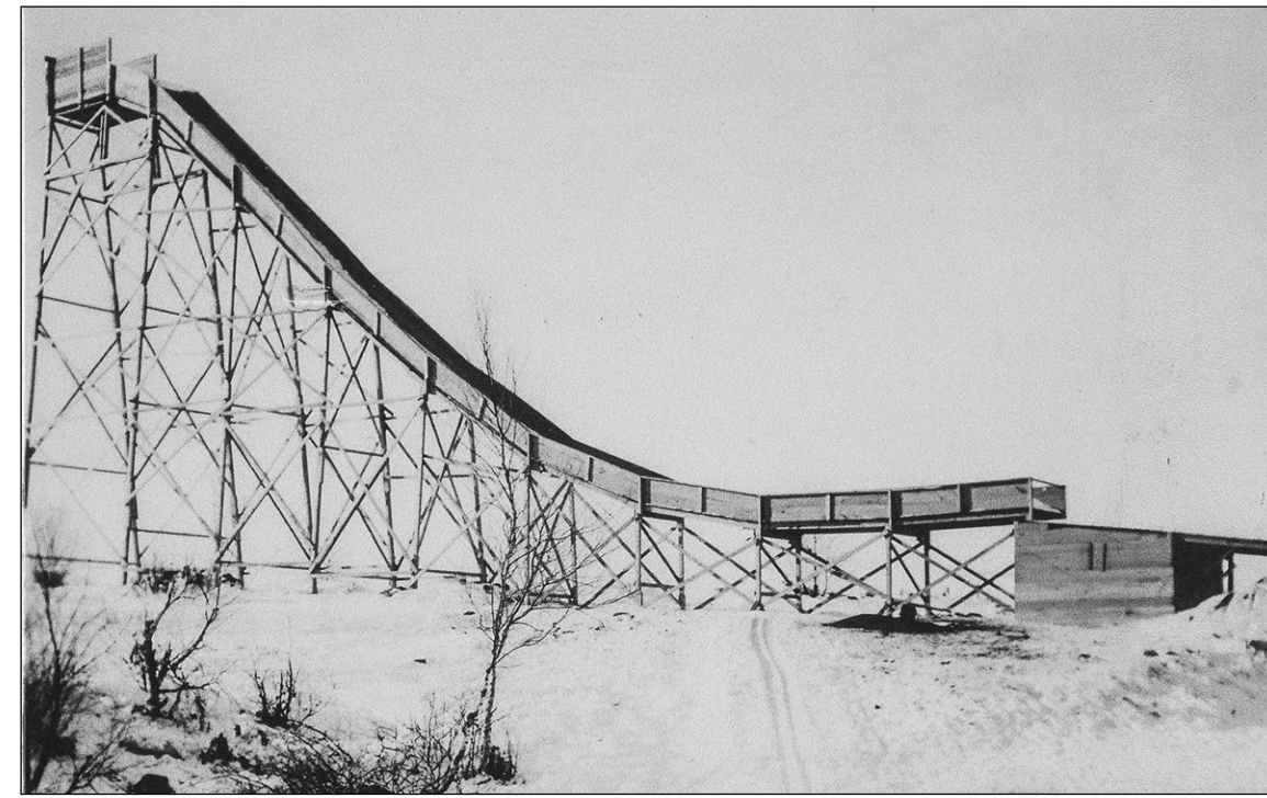
An early ski jump in Ely, on the west side of Central Ave., at a former city gravel pit at the end of W. Pattison St. The remains of the gravel pit are still there to the south of the Ely-Bloomenson Community Hospital, though the jump is long gone. submitted photo
