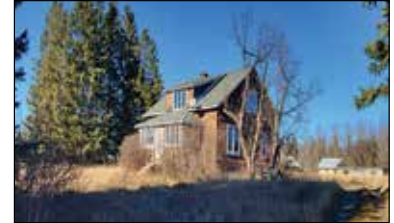
Gheen-$85,000 20-acre property with farmhouse, pumphouse, well, septic and electric. Farmhouse and outbuildings need some TLC. MLS#146075 & 6111575
