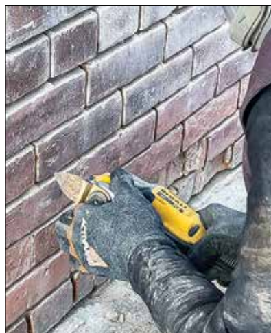
Below: A multi-tool with a pointed blade helps remove old mortar.
