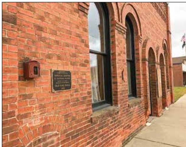
Left: The refinished front of the Old Fire Hall in Tower. Work continues on the building's interior.
