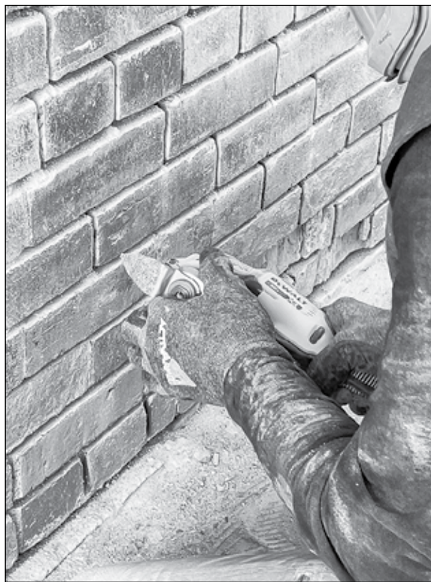
the building is complete, the next step is to work on the HVAC system and restoration and repair of the masonry on the building's interior. Plans are also
