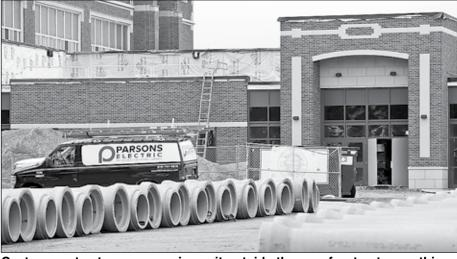
Cast concrete storm sewer pipes sit outside the new front entrance this week at the Ely school renovation project. photo by K. Vandervort
