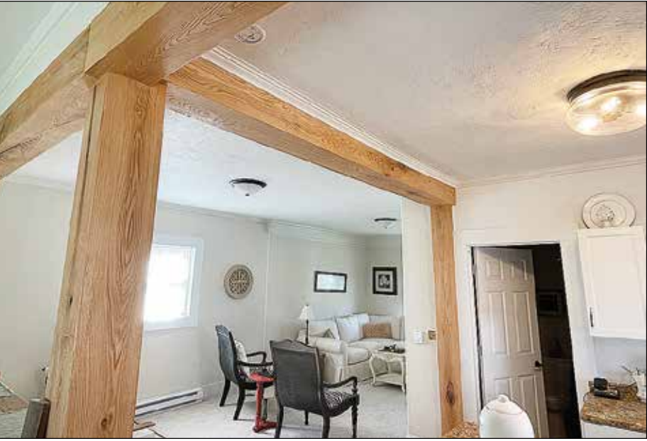
Above: The main floor in progress after plaster and lath demolition. Here, I'm sizing up the plan for removing bearing walls to replace with headers that we eventually converted into the beams, pictured at left.
