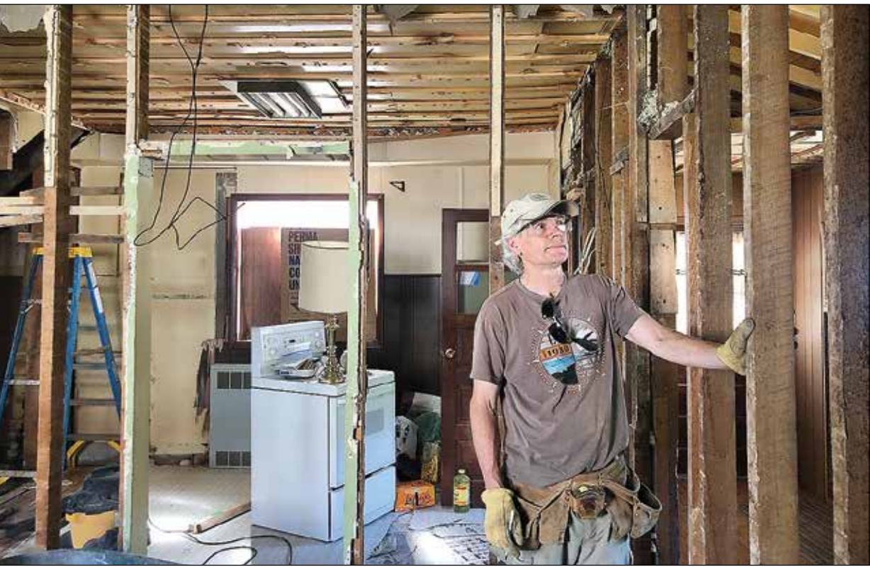
Above: The main floor in progress after plaster and lath demolition. Here, I'm sizing up the plan for removing bearing walls to replace with headers that we eventually converted into the beams, pictured at left.
