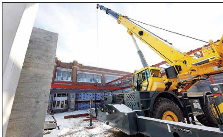
A construction crane, positioned just inside the front entrance to the new building on the Ely school campus, set roof decking this week. photo by K. Vandervort
