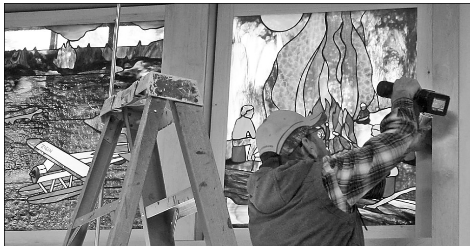
Jim Brandley did framing work on the Ely Public Library's stained glass window project to ensure the windows would be securely fastened into place. submitted photo
