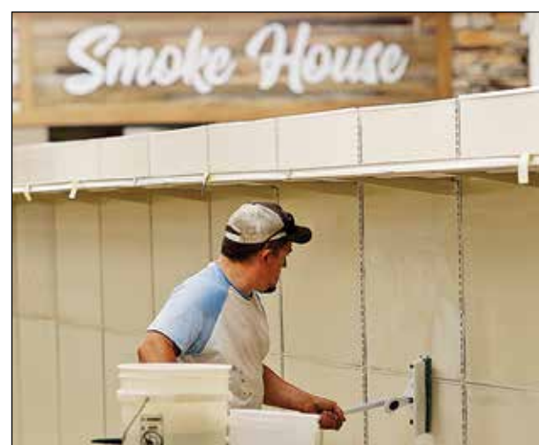
Shelving was prepared and constructed this week at the new Ely Zup's Market
