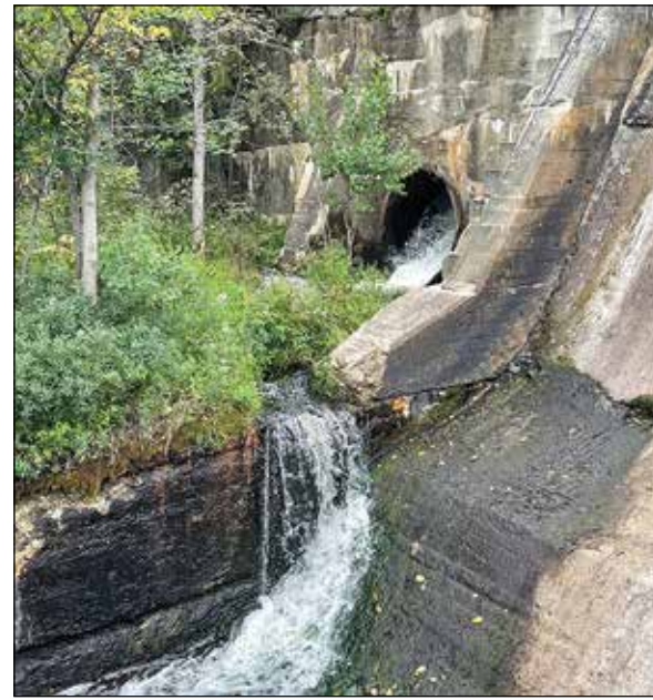
Right: The sluiceway located near the bottom of the dam continues to allow water to drain out of the flowage. Unless rain boosts river flow in the coming weeks, the flowage could actually empty.
