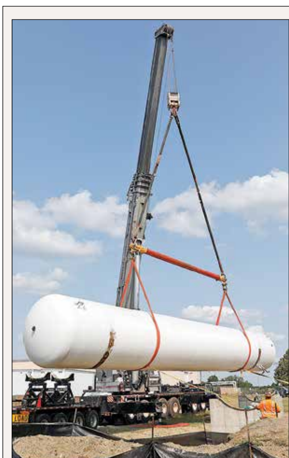
Construction crews used a specialized crane to carefully place a 60,000-pound propane tank onto a cement cradle last Thursday on the Ely school campus. The tank was relocated from the front yard of the school. photo by K. Vandervort
