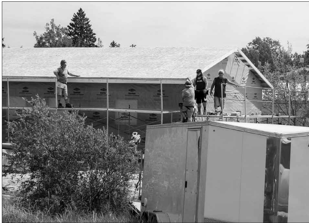
It was quitting time at the Habitat for Humanity home build on 4th Street NW in Cook on Monday as volunteers start down a ladder propped against the scaffolding. photo by D. Colburn
