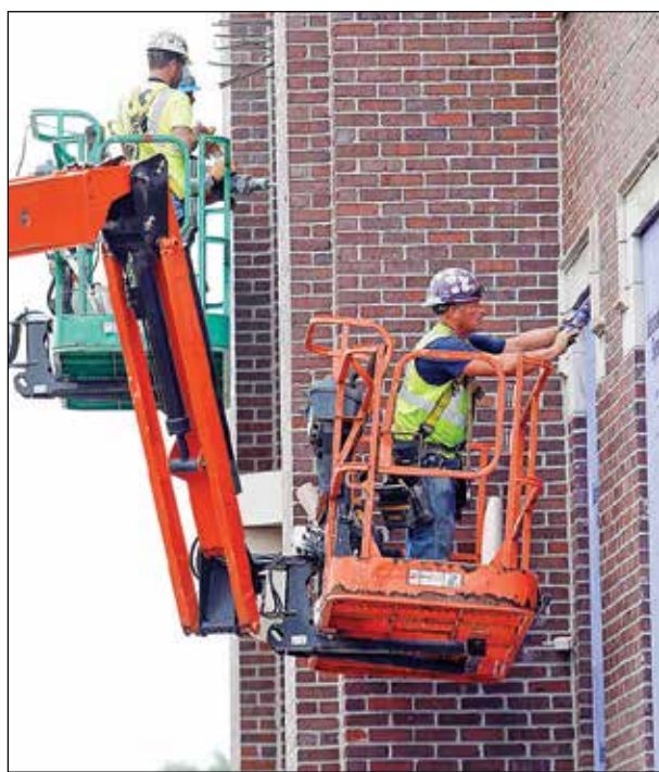
Construction crews worked on the east side exterior of the Washington Elementary building last week. photo by K. Vandervort
