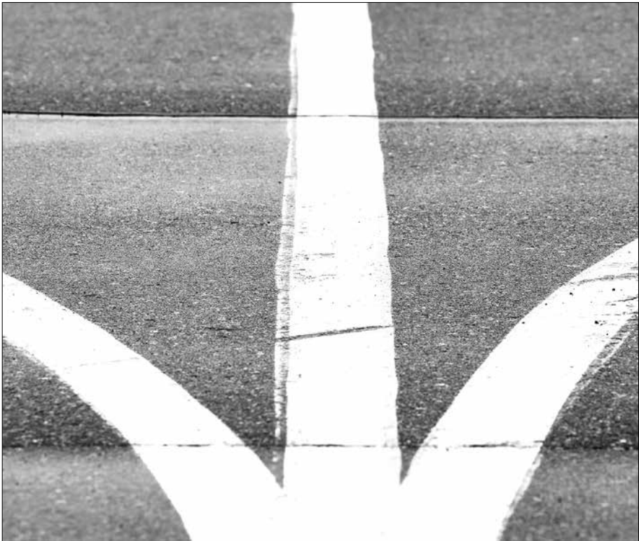
Cracks appear as horizontal creases in this picture of the taxiway at the Orr Regional Airport. A proposal to seal the cracks in the runway, taxiway, and aprons and then apply a fog seal to the finished areas is being readied to put out for bid.
