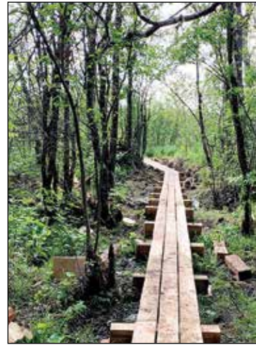
Left: The new boardwalk makes its way through a wetland as the first leg of the new Ancient Cedar Forest Trail now under construction in Tower.
