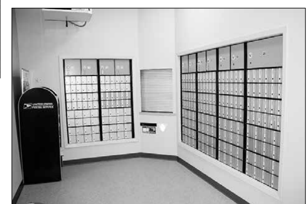
The building remodel also included lots of new improvements to the Soudan Post Office, which leases space in the building. The post office now features keyed locks and a remodeled entrance and lobby area.
