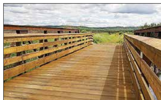
A new bridge at the Darwin Myers Wildlife Management Area in Embarrass is now completed. Courtesy MNDNR
