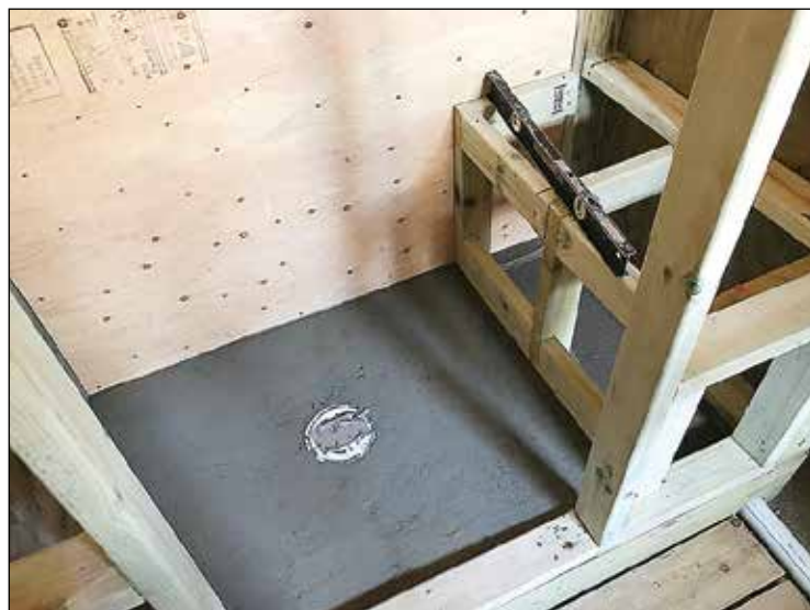
Above: The stall and bench framed in and the first layer of dry-packed mortar in place. The mortar should be flush with the first part of the two-part drain system. You'll screw on the second part of the drain once the mortar is set.
