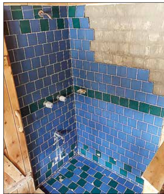
Below: The original shower, with chipped tile, in desperate need of replacement.
