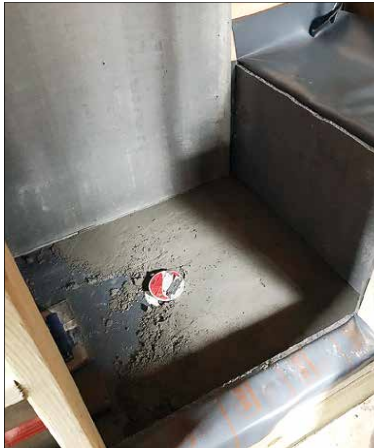
Above: The stall and bench framed in and the first layer of dry-packed mortar in place. The mortar should be flush with the first part of the two-part drain system. You'll screw on the second part of the drain once the mortar is set.
