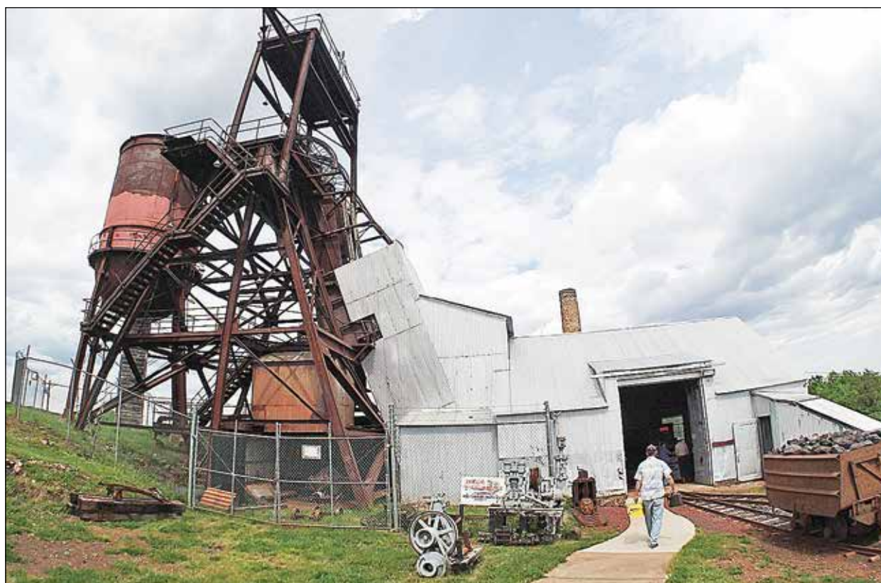
The city of Ely was granted a $10,000 Minnesota Historical and Cultural Heritage grant to assess the condition of the Pioneer Mine site. photo by K. Vandervort
