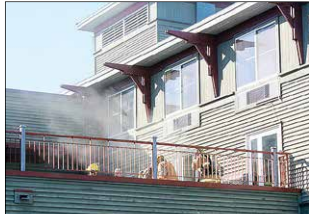
The fire was contained to a single room on the fourth floor, but smoke permeated through other parts of the hotel. photo by Max Helmsberger
