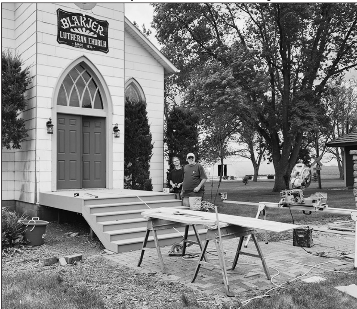
Blakjer Church, in Lone Rock, has undergone an impressive renovation. New entry steps were installed by Todd Gifford of G&G Construction. Respectfully Submitted by Letty Henriksen, Lone Rock Correspondent
