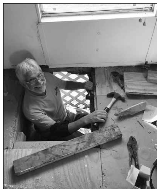
Kirk Chamberlain volunteers with the COA by helping with home repairs.
