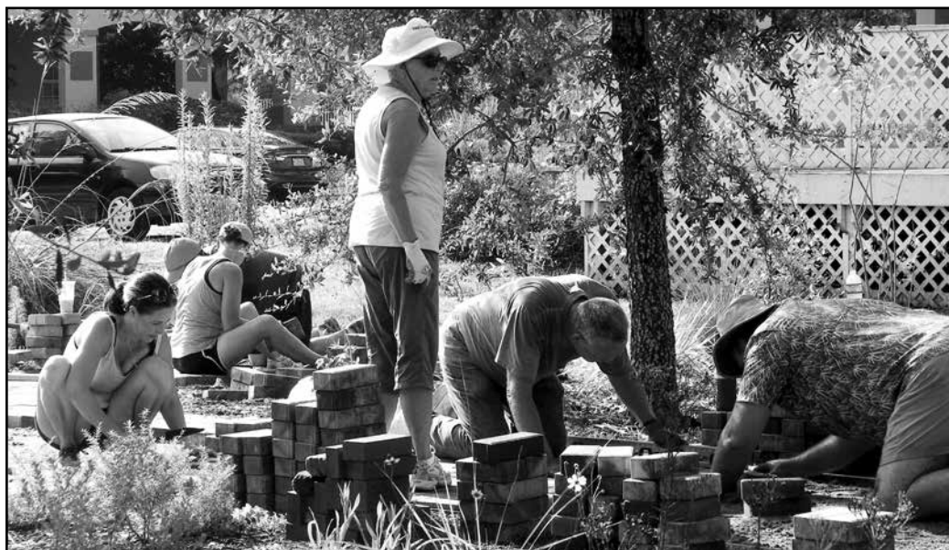
A group of COA volunteers installs pavers.
