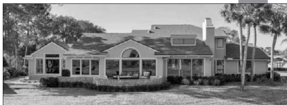
The back of the property is displayed after renovations.
