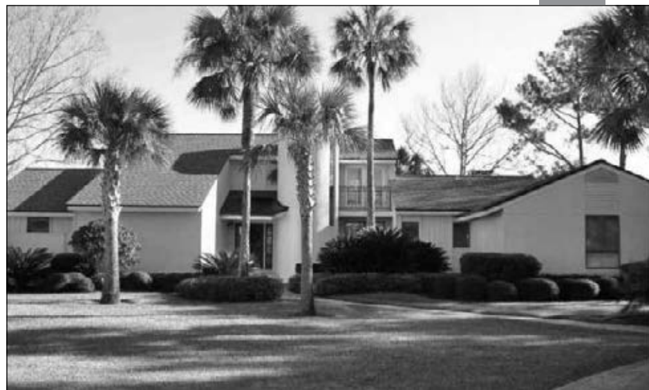
9449 Preston Trail West stands before renovations.
