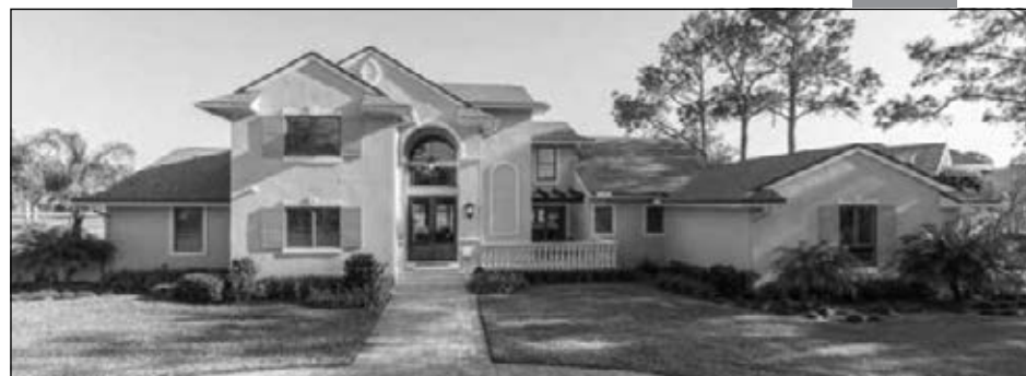
9449 Preston Trail West stands after renovations.
