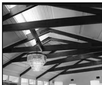
ABOVE: Ceiling panels were implemented to reduce noise in the restaurant.
