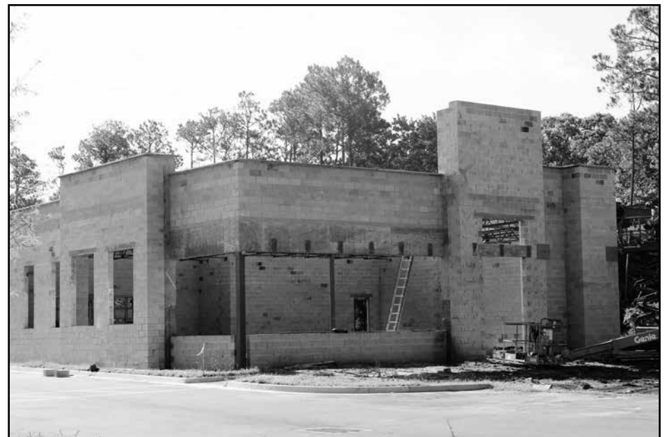
Crosswater Dental Care under construction
