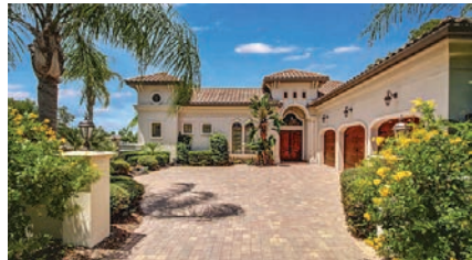
Enchanting Italian Courtyard Custom Home Constructed by Elwood Collier in the exclusive Pablo Creek Reserve. If you are looking for an open floor plan, you have found it! Huge wooden doors open to spacious courtyard featuring a summer kitchen and heated salt water pool/spa lit by two gas "coal pits." Courtyard connects to the guest house complete with mini-kitchen and master suite. All three bedrooms on the property offer luxurious ensuites. $1,055,000
