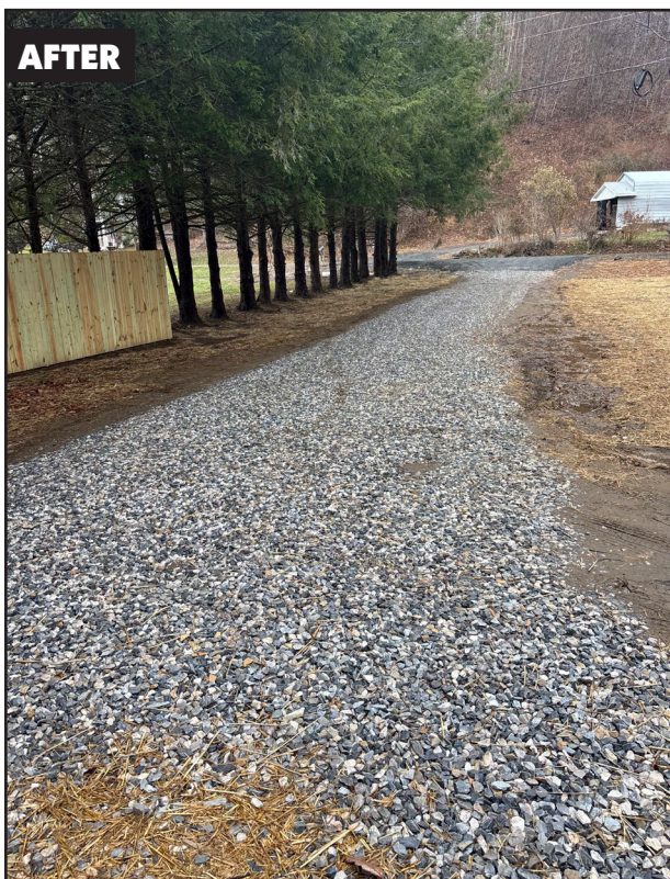
After paving a gravel driveway
