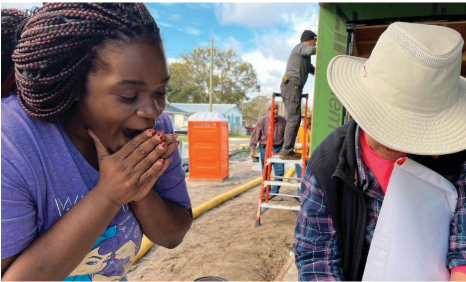
A new homeowner, identified only as Antwoinette, reacts joyfully to work being done on her home.
