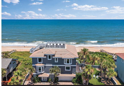
And aerial view of the front of the home.
