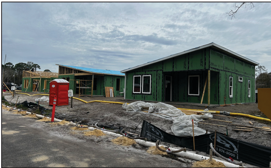
The first three homes are under construction in Volusia Woods.
