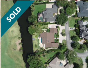
3255 Old Barn Road West
