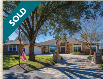
3253 Old Barn Road West
