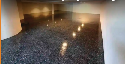
3D Metallic Epoxy Flooring
