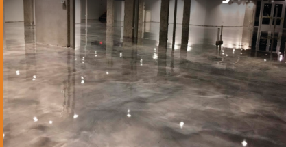
Concrete Polishing
