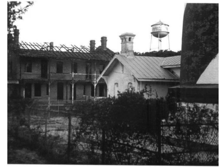
The roof being repaired on the Keeper's House.
