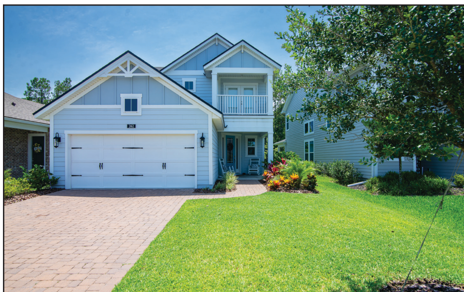
The home at 262 Pioneer Way Drive.
