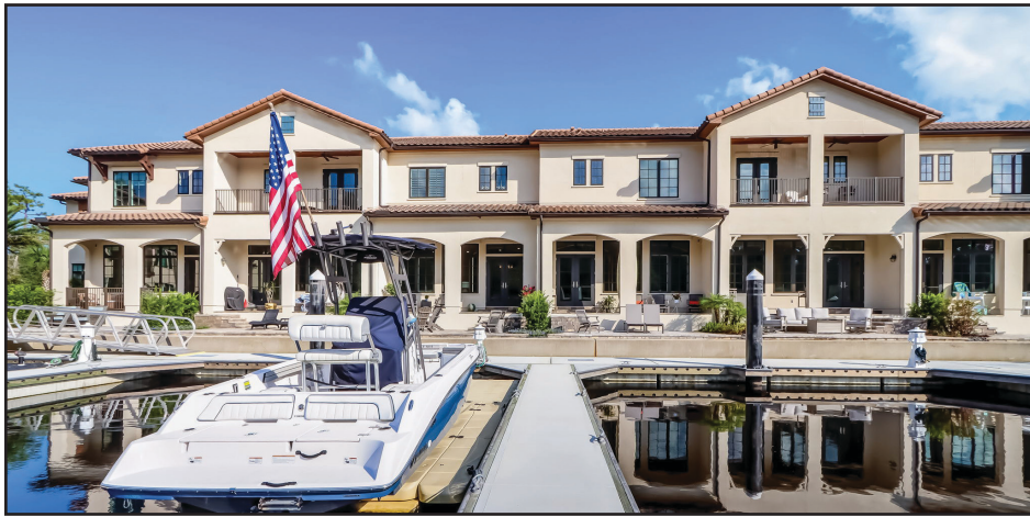
The two-story coach home has two 50-foot boat slips.
