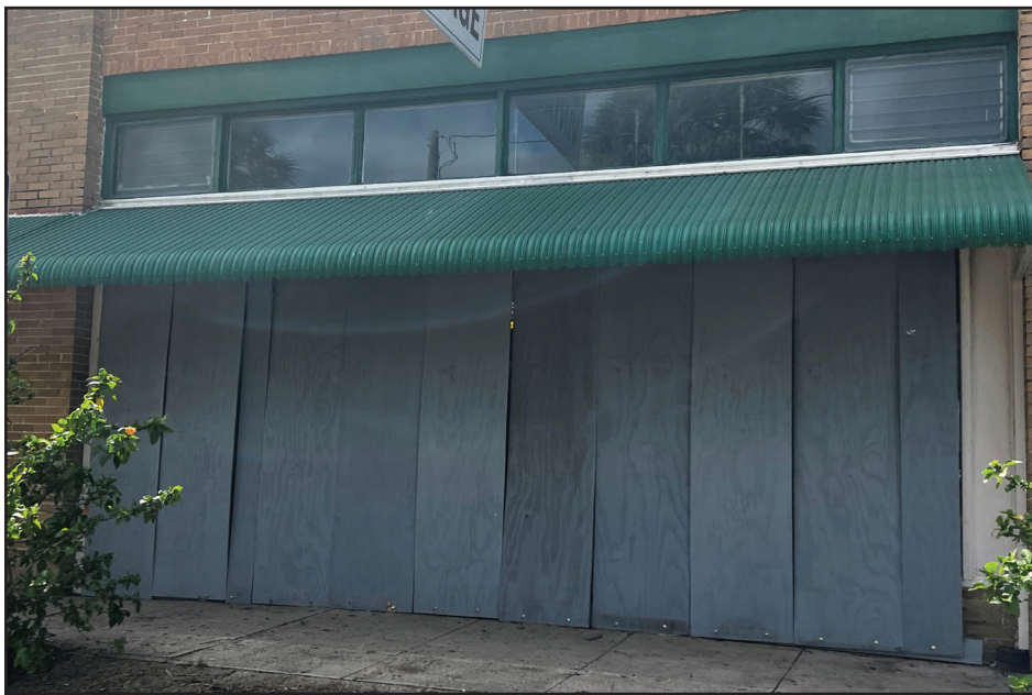
St. Augustine businesses boarded up their storefronts to protect them from the storm.
