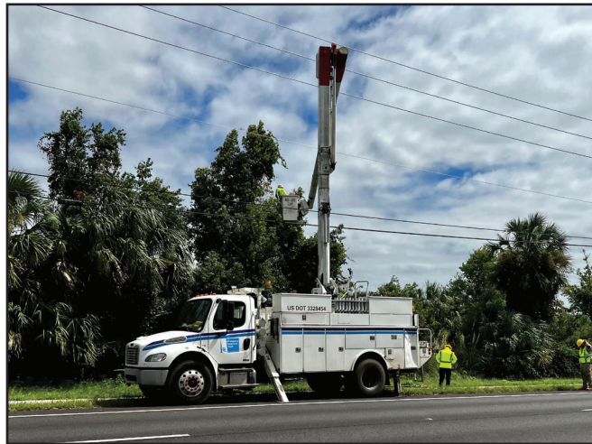
Utility crews were out repairing lines after the storm had passed.
