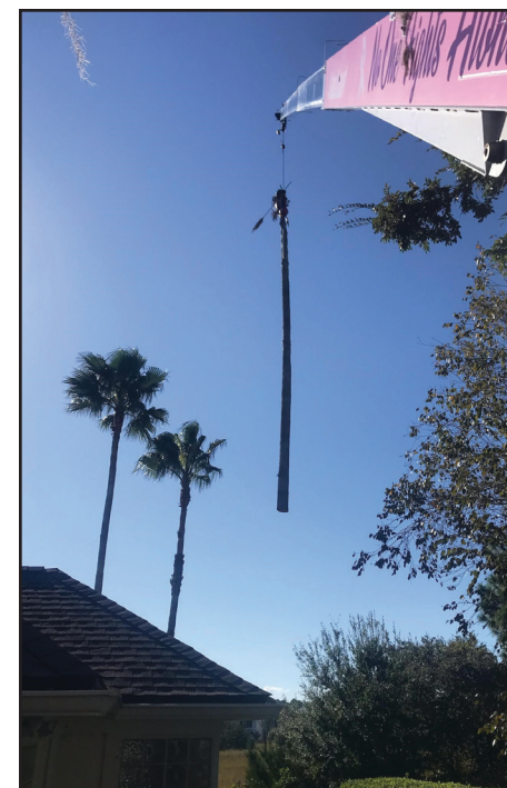
A 110-foot crane removing a 50-foot palm tree off a house.
