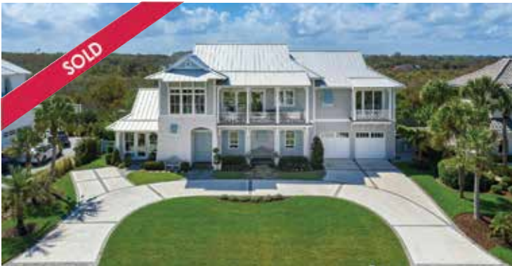
Sophisticated Coastal Luxury A masterpiece of design and craftsmanship, this custom beach home was thoughtfully designed by Nesting Place Interiors 7 Heritage Homes and offers a neutral coastal palette with panoramic views of the Ocean and Guana. 4 bedrooms, 3F/2H bathrooms
