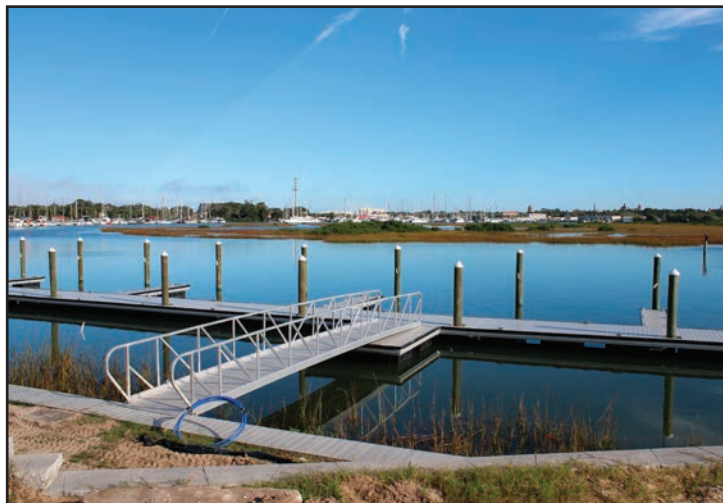
Adjacent boat slips included in the purchase price can accommodate a 40- to 70-foot boat with water and electric provided.
