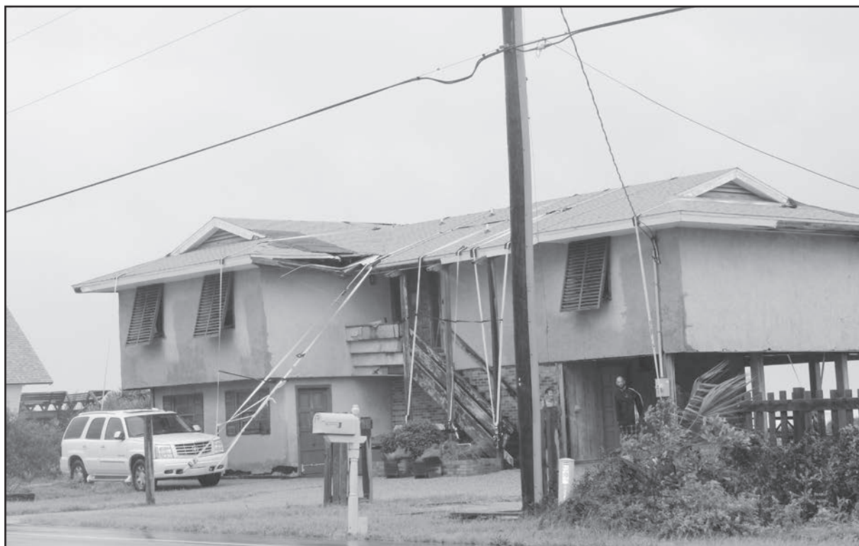
In an effort to save the structure, residents used tie-down straps over this home in South Ponte Vedra on A1A. Some of the straps are attached to fixed objects; others are attached to the Escalade in the driveway.
